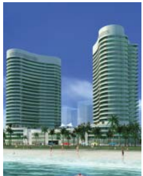
The Beach Towers project is expected to be complete by mid 2010.
